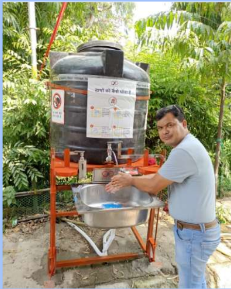
Handwashing station installed at Kalyanpuri police station main gate in east Delhi
