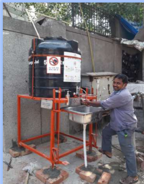
Handwashing station installed in front of Kali Mandir, Jasola village in south-east Delhi
