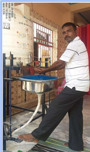
Handwashing station installed at Block 33, Trilokpuri in east Delhi
